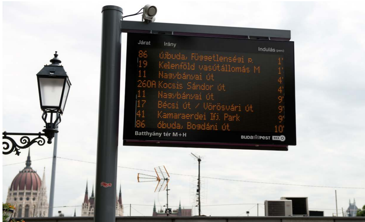
The VECTOR system provides up-to-date arrival times. Thanks to a newly invented info terminal, it even works without external power sources. Travelers use a crank which generates electricity. The terminal then shows transport information on an e-ink display in real-time.
